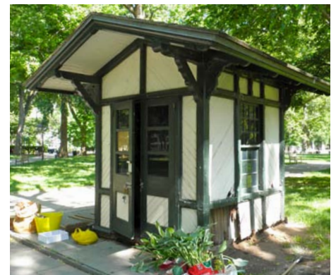
The southeast shed (pictured above) has been removed for repairs. The northwest shed will be repaired in place.
