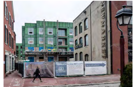
Toll Brothers construction at the New Market site.
