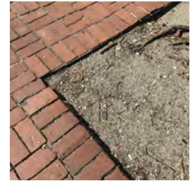
This flat edge is the best way to fix your tree pit and allow rainwater to drain into the soil.
