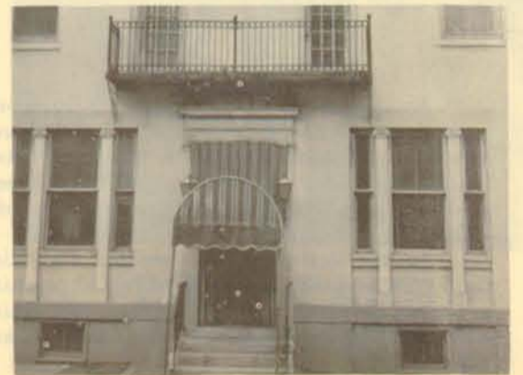
Portion of the building at 431 Pine Street that would house the proposed Washington Square Theater
