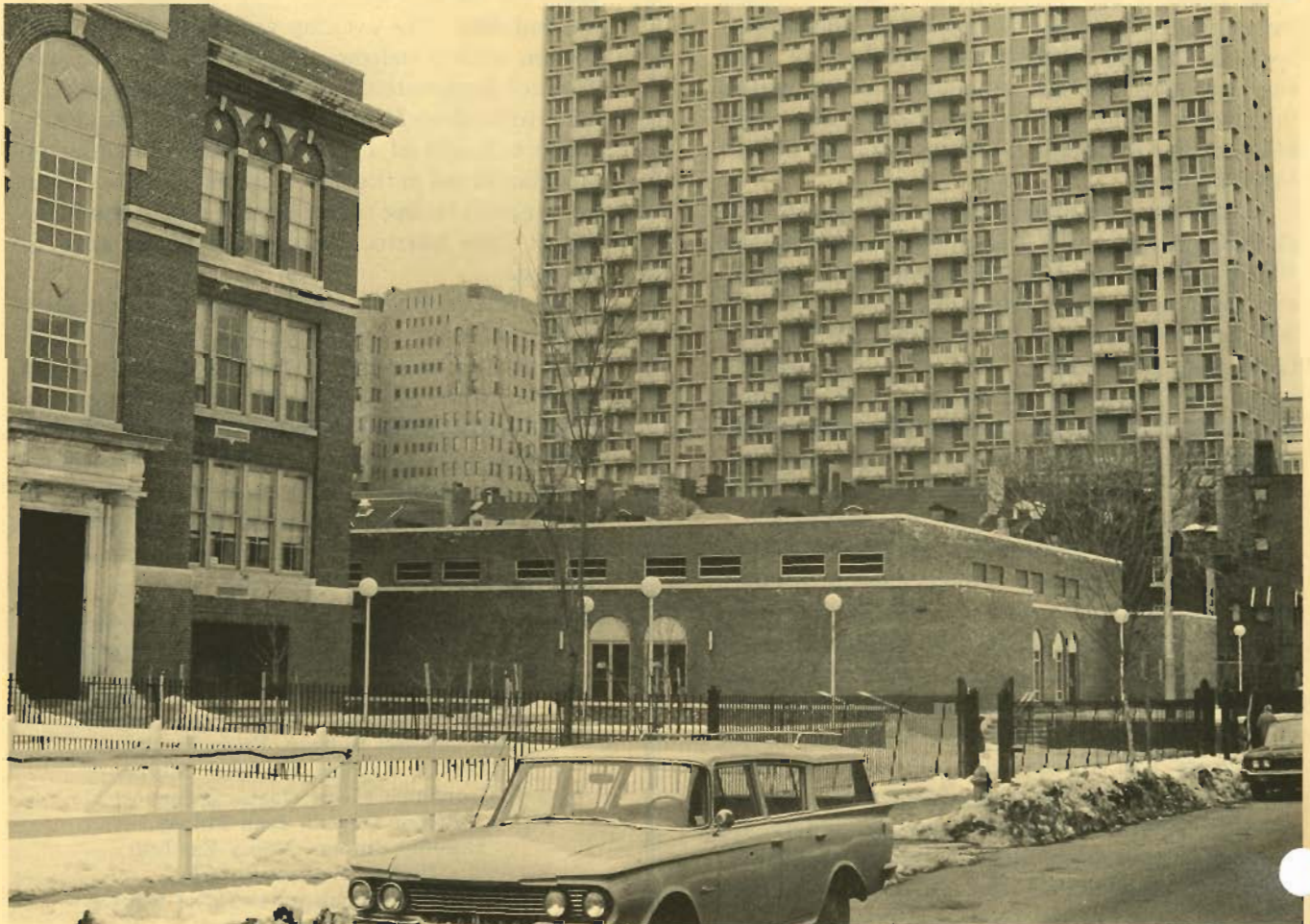
New gym-auditorium, a handsome addition to recently renovated 1907 school building.
