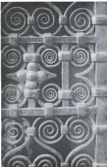
Detail, gate at entrance to Lea & Febiger; Samuel Yellin.
