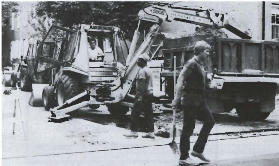
Where crews dig on Spruce Street,
