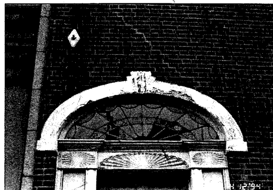
This York Row house fanlight will be restored and preserved.
