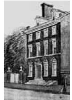
When Philadelphia was capital of the U.S., first George Washington and then John Adams occupied this house at 190 High (Market) Street.
