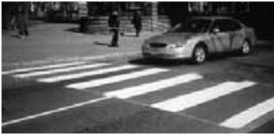
Newly painted crosswalk should improve pedestrian safety at 6th Street and Independence Place.
