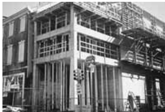
Construction is well underway at York Row.
