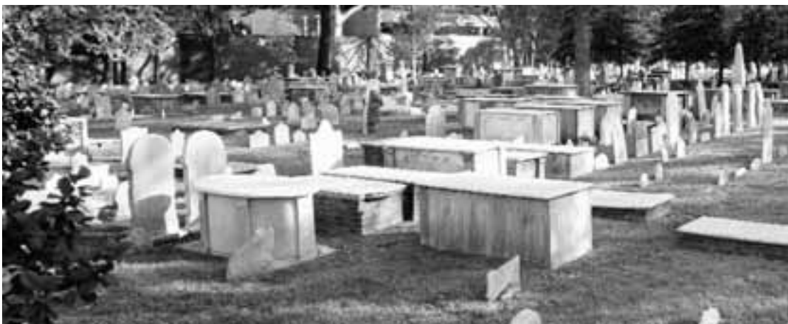
The Old Christ Church Preservation Trust raised the funds to repair graves and markers, rebuild the wall around the cemetery and landscape the grounds
