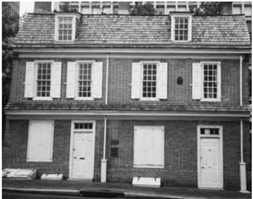
The Man Full of Trouble Tavern is sporting a new cedar shake roof.
