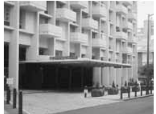
Hopkinson House was the first residential high-rise built in Society Hill.
