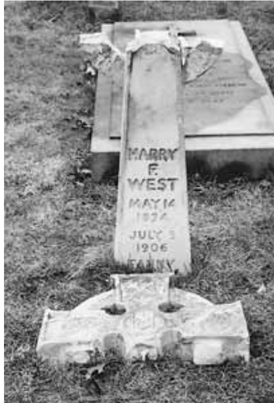
A CRYING STONE: This recently vandalized grave marker with the top knocked off is one of five broken since December. It will be repaired this year by John Carr.
