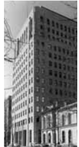
The N.W. Ayers Building photo from the Bernie Cleff Collection, Athenaeum of Philadelphia
