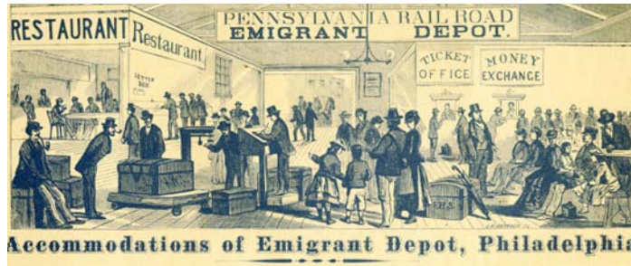
Accommodations of Emigrant Depot, Philadelphia Interior of the Washington Avenue Immigrant Station (Pennsylvania Railroad Emigrant Depot), circa 1885. Image courtesy of Independence Seaport Museum (Philadelphia, PA), 1965.217.
