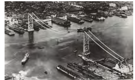
The Ben Franklin Bridge, then known as the Delaware River Bridge, under construction.
