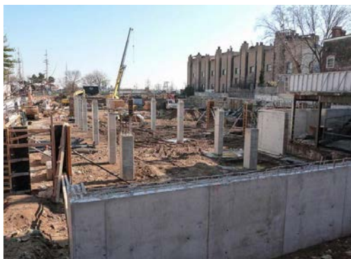
Project construction progress as of December.
