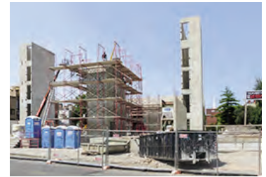
Construction is progressing at the Toll Brothers 410 South Front Street site.
