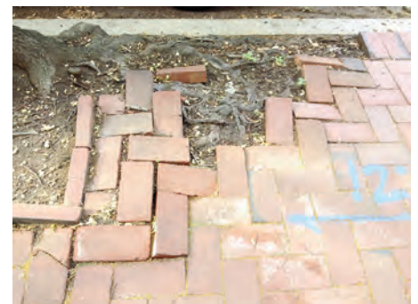
If tree roots are dislodging bricks on your sidewalk, get estimates for repair.
