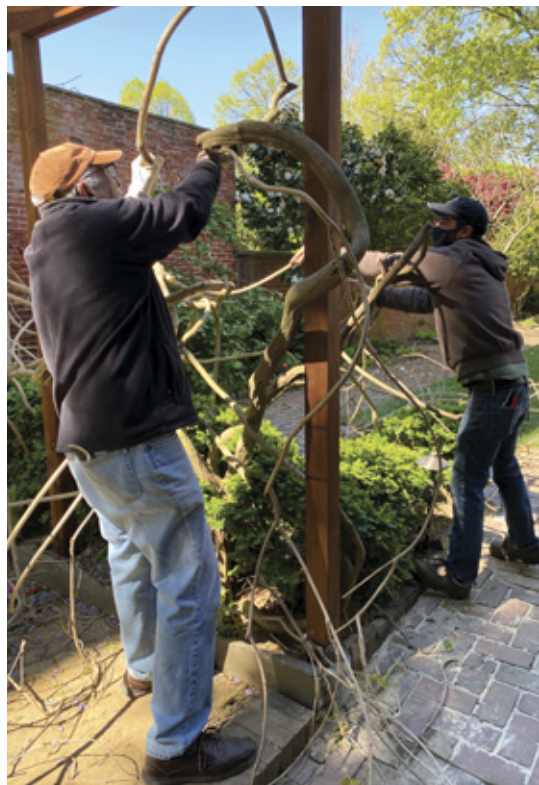
Vines are wrapped around the new trellis.
