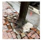
This poor tree needs its pit to be expanded with a defined surround, one that is flat to avoid trips.
