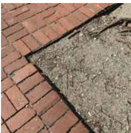
This flat edge is the best way to fix your tree pit and allow rainwater to drain into the soil.
