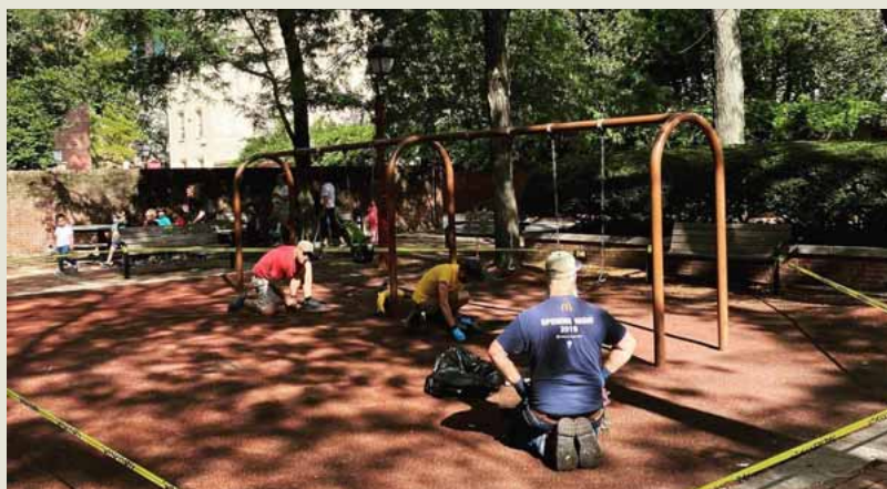
Workers completing surface repairs to the playground at Three Bears Park.
