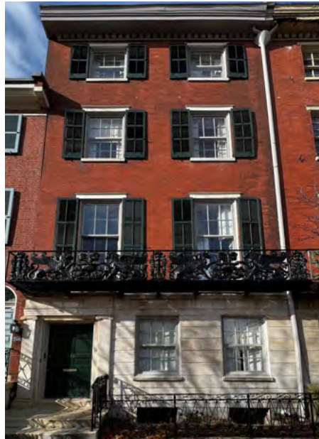
234 S. 3rd Street after exterior restoration was completed.
