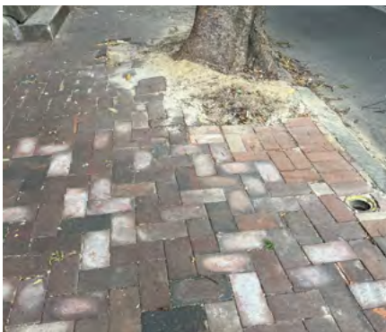
Bricks replaced after many complaints to the Water Department.
