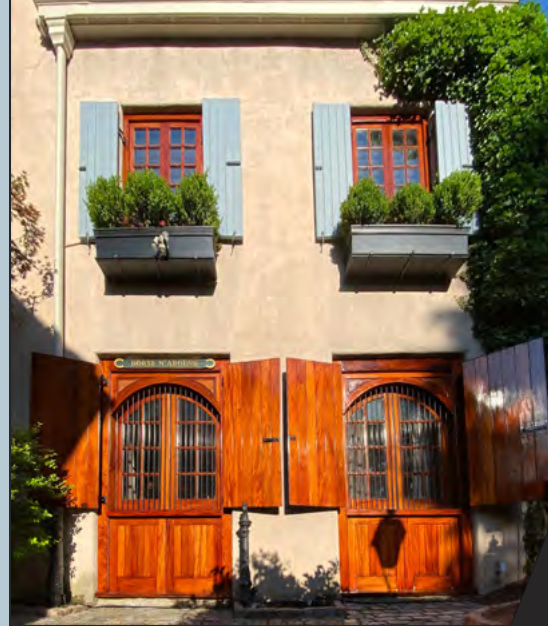
Our Historic Restoration of a Horse Stable Home in Society Hill
