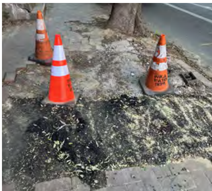
Spruce Street Water Department excavation site.
