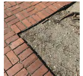
This flat edge around a tree pit allows rainwater to reach tree roots.
