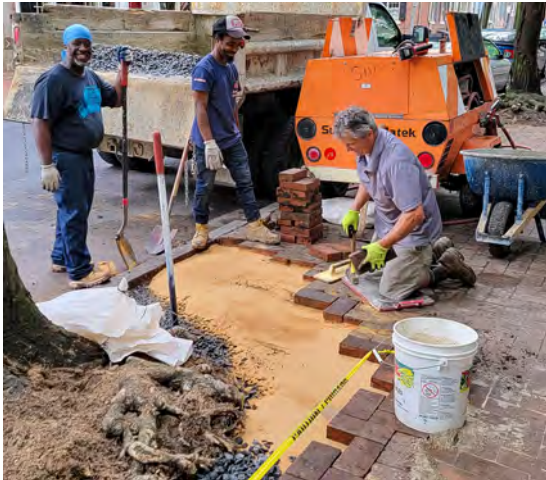
Contractors resetting bricks to level a sidewalk.
