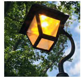
High pressure sodium bulbs emitting warm light are slated to be replaced with LEDs as part of a citywide energy saving project. The City of Philadelphia and the Philadelphia Energy Authority have launched trial installations for the Philly Streetlight Improvement Project, a comprehensive LED streetlighting, controls and networking project.
