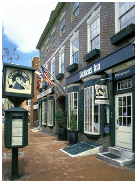
The Dickens Inn, 421 South 2nd Street
