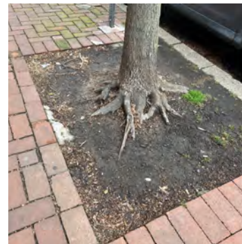
Excellent tree pit: right size with flat edge allowing rain water in.
