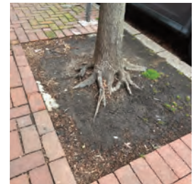
This is the ideal tree pit. Flat edges let rainwater flow into the tree pit. There are no loose bricks to tempt vandals.
