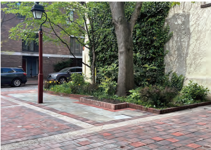
Completed restoration work
