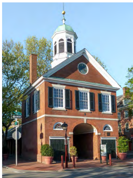
The Foundation provided funds to the Conservancy to make repairs to Head House and the iconic Lukens clock.
