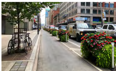
Planter separated bike lanes in Toronto
