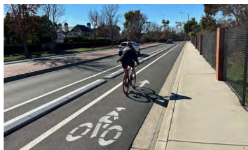
Concrete-protected bike lane in Long Beach
