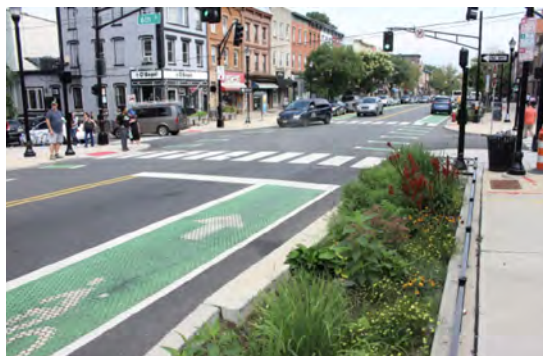
Hoboken corner with a bump-out curb planter
