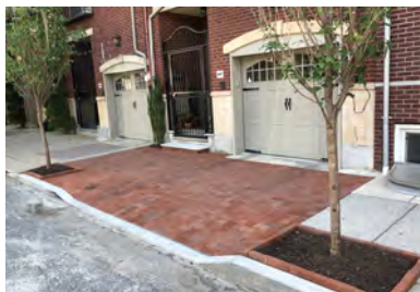
Fix your Bricks. Society Hill sidewalks should provide smooth, safe walking surfaces. The upheaval caused by tree roots can be corrected without removing or killing trees. Call McFarland to inquire about fixing your bricks.
