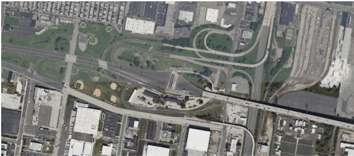
Figure 8 Existing Walt Whitman Interchange (I-95 at I-76) base source: Apple Maps, OpenStreetMap.org
